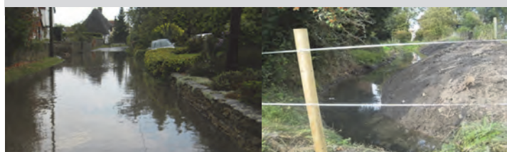
York Road flooded from end to end and the newly cleared ditch
